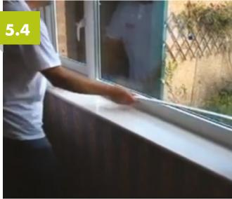
Make sure the area is clean and free from dust and debris. Measure and fit any internal trims that may be required. Trims maybe fitted using a suitable PVC-U adhesive or silicone.
